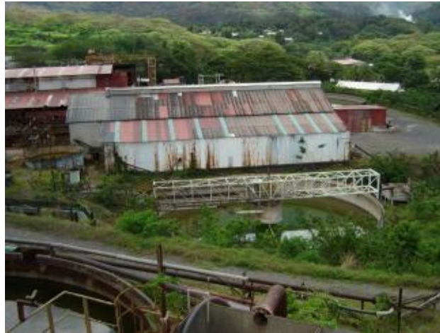
30 m crusher slimes thickener
