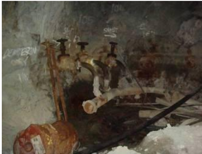
Dewatering Holes - R1/Cayzer Decline 17 Lev
