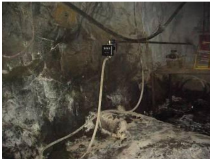
Diesel Bay – Smith Shaft
