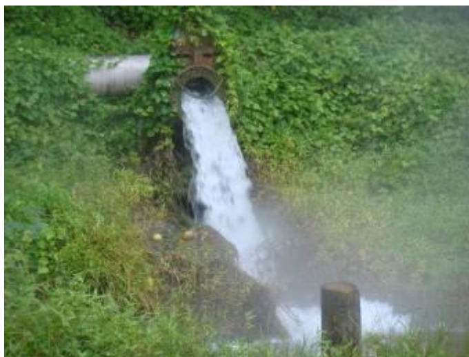
Dispersion of Fissure Water Pumped Out of Cayzer Shaft
